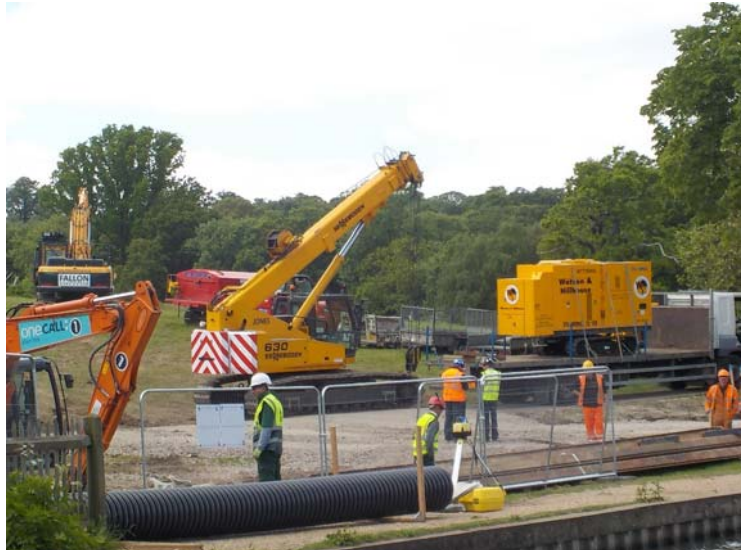
Picture 4 - Forty ton crane being used to move sheet metal piles into place.
