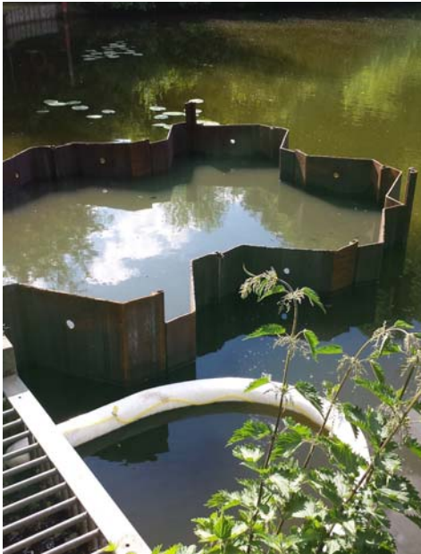
Picture 7—Temporary coffer dam at Viaduct Pond
