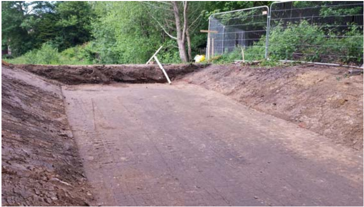
Picture 8—Spillway under construction at Viaduct Pond.
