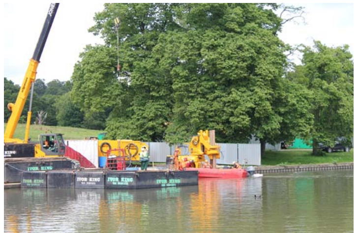
Picture 6 - The piling rig pushing the sheet-metal piles into place using a silent vibration-less technique.
